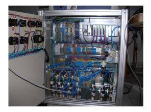
Fig. 1 Interior of an evaporator leak tester with cRIO controller
